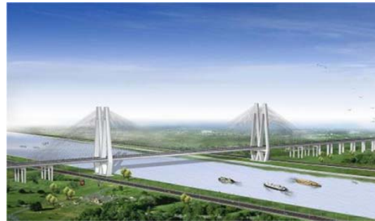
Ningbo Yongjiang Grand Bridge Zhejiang Province, China
