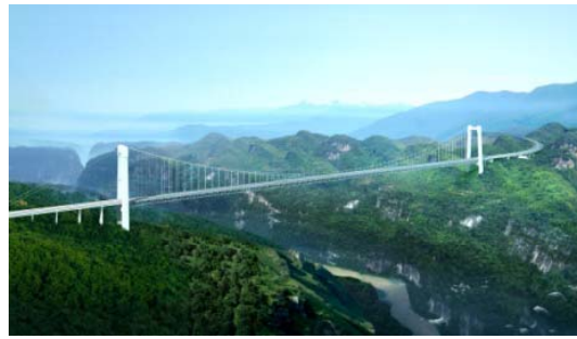
Lishui Grand Bridge Hunan Province, China
